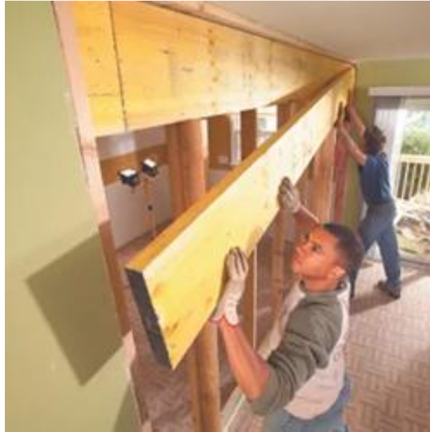
Adding a huge load-bearing beam to open an interior space
