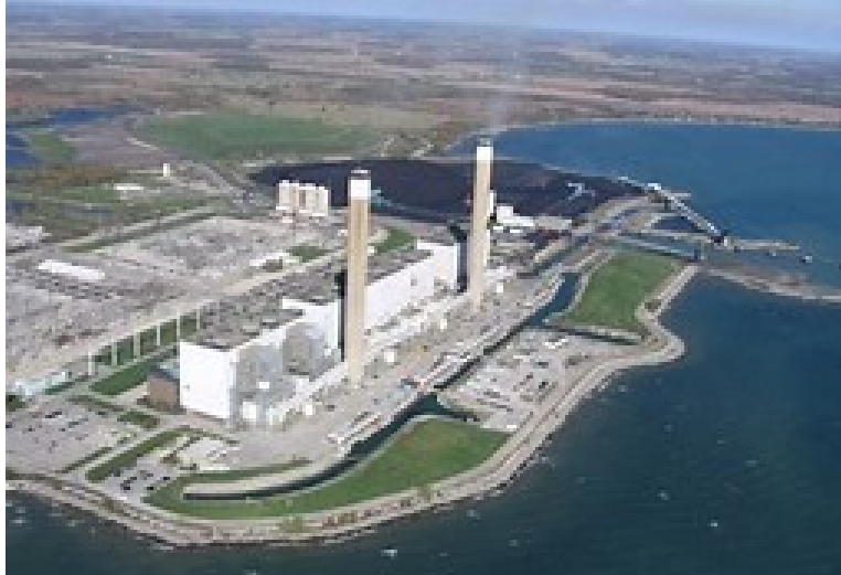
The former Nanticoke, Ontario Power Plant with its distinctive 650-foot smokestacks could be seen from the ridges south of Erie on clear days.
