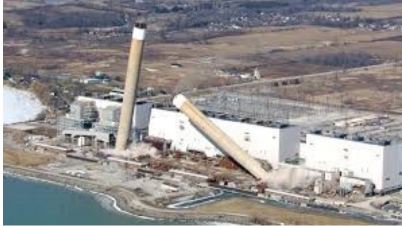
The twin 650-foot stacks are brought down at Nanticoke.
