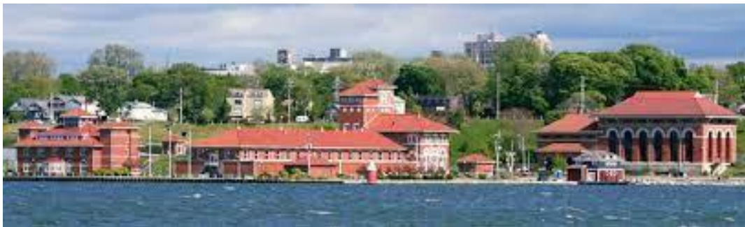
Erie Water Works bayfront campus
