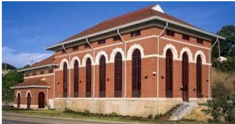
The building that houses Big Bertha
