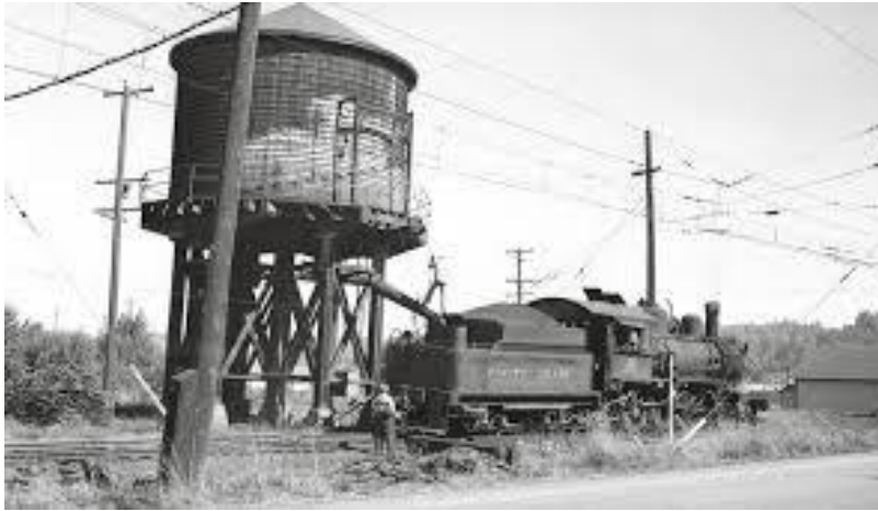
A vintage steam locomotive being gravity-filled with water at a water tank
