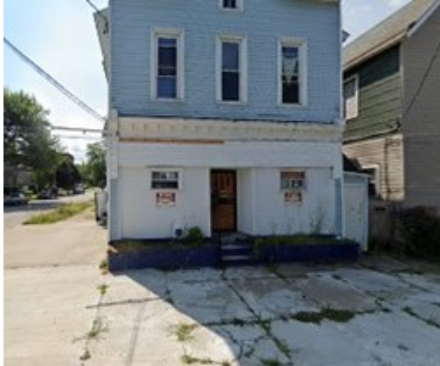
The current Star Lite Hotel building, complete with bullet holes, is out of business, boarded up, and suggesting that the anti-neighborhood hotel movement of the 1970s wasn't a bad idea.
