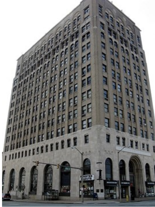
The Erie Trust Building became the Baldwin Building in 1943 and later the Renaissance Centre.
