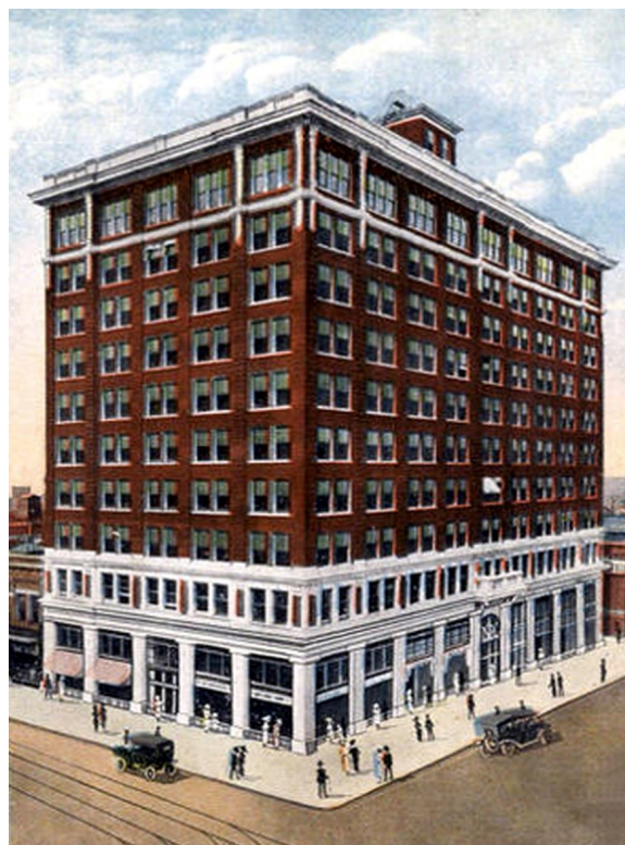
The Commerce Building, Erie's first skyscraper.
