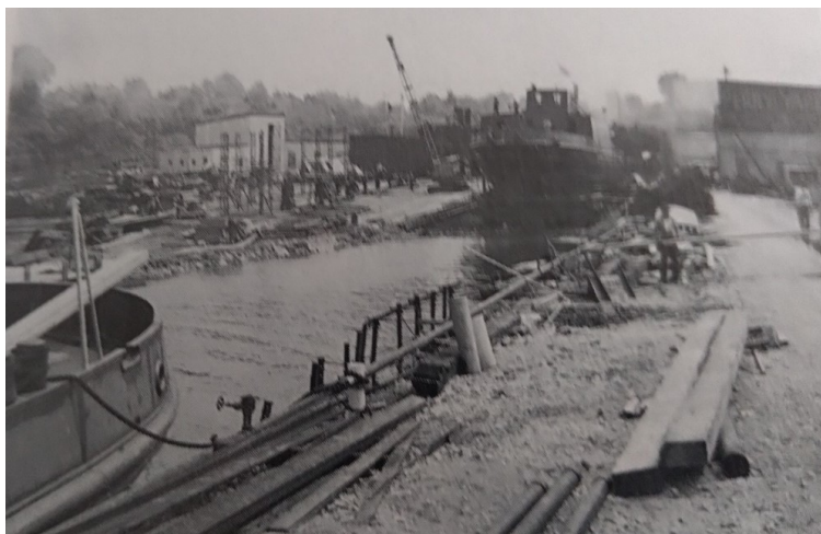
Our 1950s fishing emporium looked more like an ugly industrial site than a lovely fishing hole. Rusty pipes and beams, ancient boat hulls, derelict railroad ties, and other random detritus littered the area for decades.
