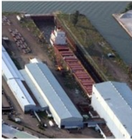
Erie's Donjon Shipbuilding & Repair facilities with a 1,000-foot ship in the drydock
