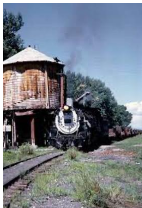
Typical steam engine water tank
