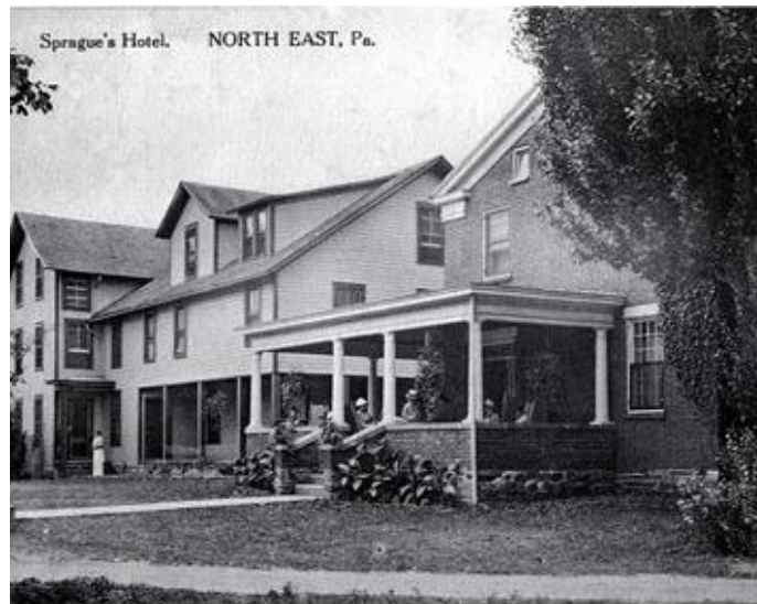
The Sprague Lakedale Hotel complex is shown in about 1920. The brick building at right is the original 1835 house and tourist home while the larger structure at left is the 11,000-square-foot hotel.
