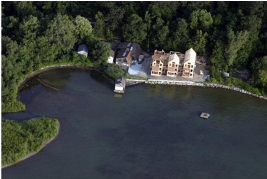
This ten-year old view of Dave Bierig's sail-making shop shows modern homes on his right under construction and a small cottage on the left, all at the outflow of Cascade Creek. Bierig's Sail Making Loft, designed by his architect wife, Susan Sprague, is in the center. The original Finn Yacht Club was in his current parking lot to the right of his buildings, and the second club was on the left just beyond where the cottage is now. (Photo by Jerry Skrypzak from a plane piloted by Tom Zawistoski)
