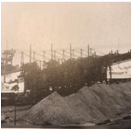
The eastern (Carnegie) dock is shown in the foreground with the middle dock in the background. Note the row of Brown hoists.
