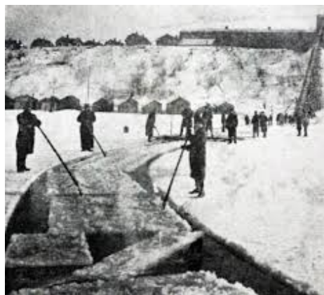
The winter ice harvest took place on Presque Isle Bay. Note the elevator on the bluffs, lifting slabs of ice up to an icehouse.
