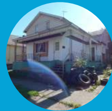
Photos of blight and decay in Erie County.
