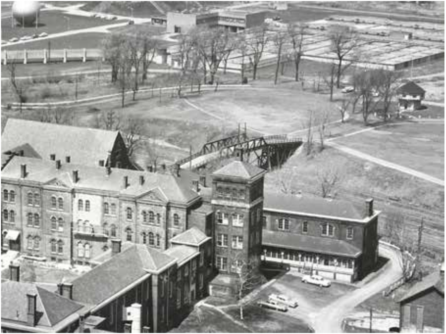
Figure 23. Pedestrian bridge connects Wayne Blockhouse to Soldiers' & Sailors' Home over railroad tracks, circa 1960.
